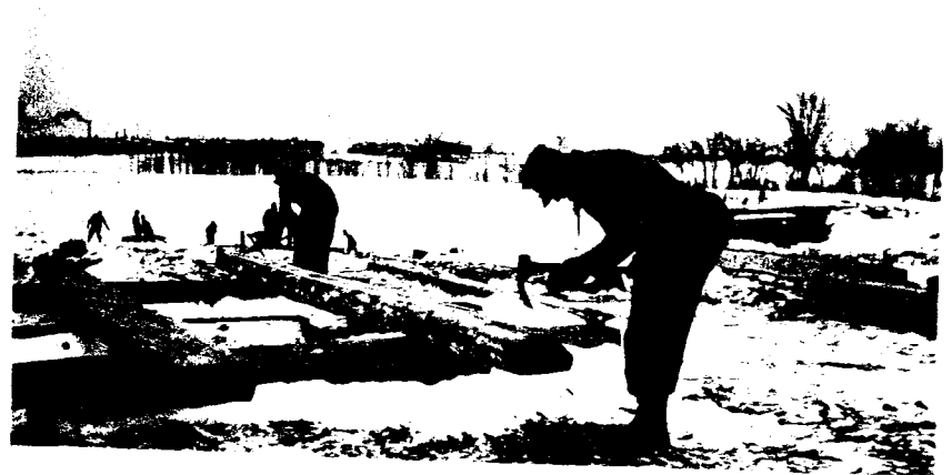
Photo. # 14. Project 1016-B; - Framing logs - Adze work.
