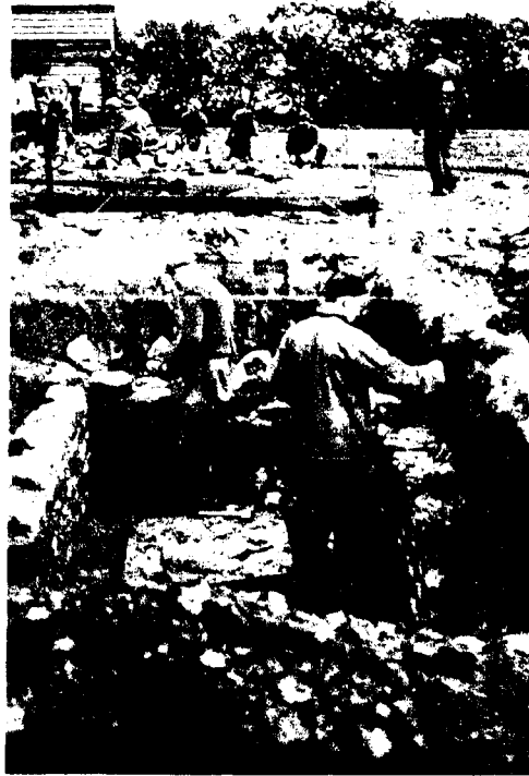
PROJECT 1016A FOUNDATION RESTORATION ISAAC GOLLIHERS RESIDENCE AND COLD CELLAR SHOWING CELLAR
