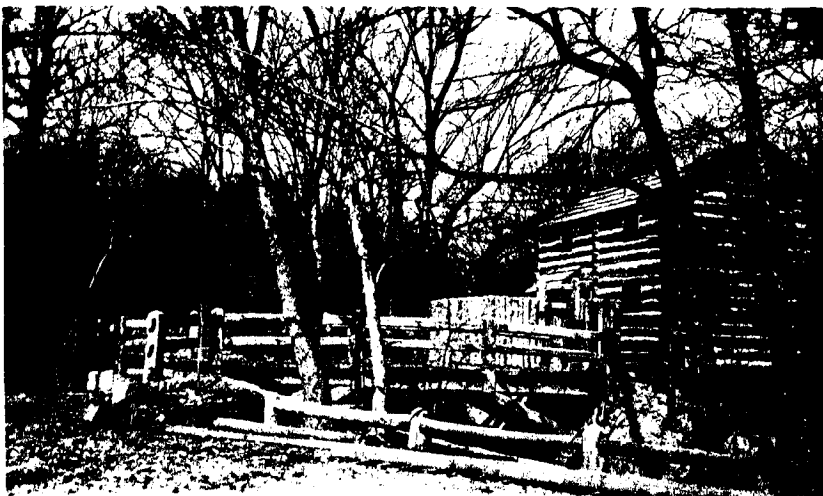
Photo. # 6. Project 101 - Footbridge to Tavern looking west.
