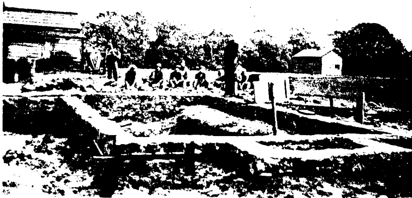
PROJECT 1016A FOUNDATION RESTORATION ISAAC GOLLIHERS RESIDENCE AND COLD CELLAR SHOWING RESIDENCE
