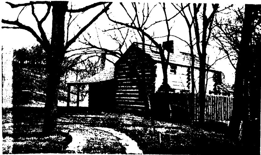
Photo. # 7. Project 702-A Fine grading at Tavern looking northeast.
