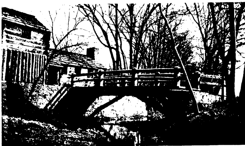
Photo. # 11. Project 101 - Footbridge to Tavern looking northeast.
