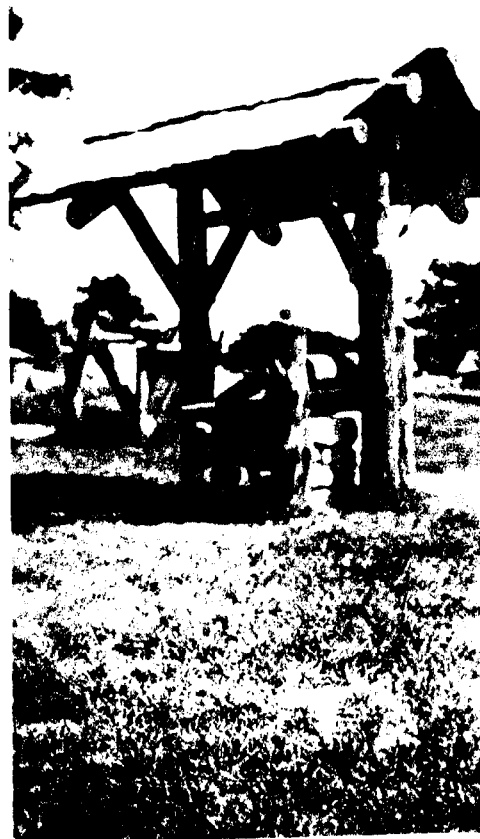
Photo. # 10. Project 1016-C - Peter Lukin Well.
