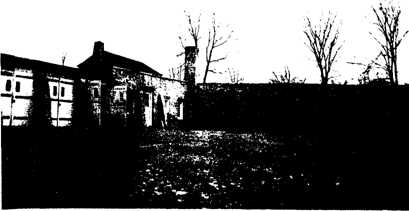
Photo. # 4. Project 108-B - Service area and Building looking northeast.
