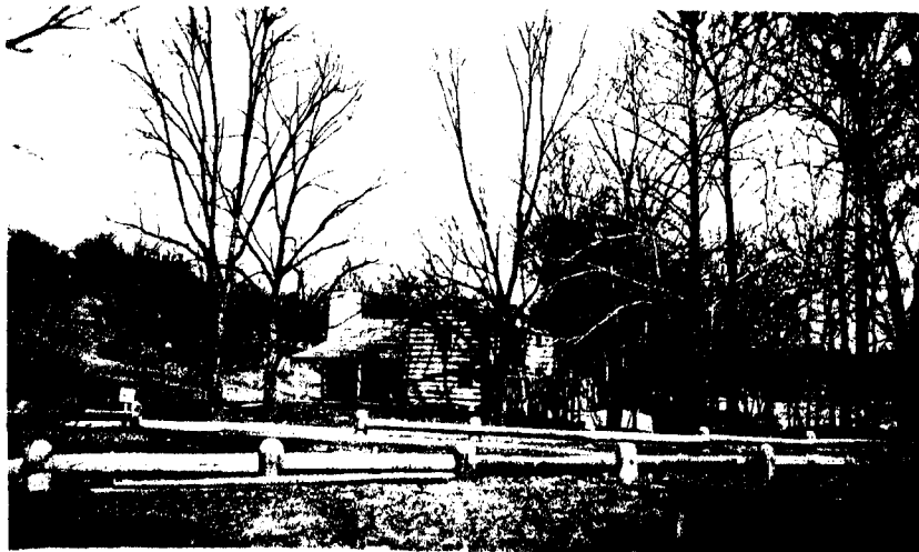
Photo. # 9. Project 108-C Tavern and comfort Station looking East.
